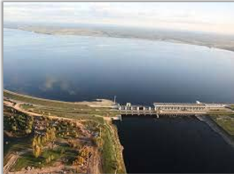
Riga's water reservoir (Source: Latvenergo.lv)
